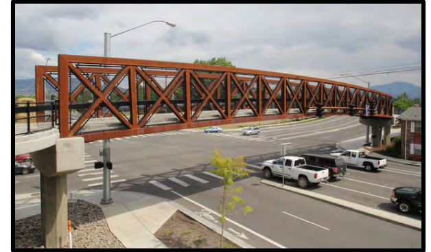
6: PEDESTRIAN BRIDGE ON SR 54 TO MCCURRY PARK
