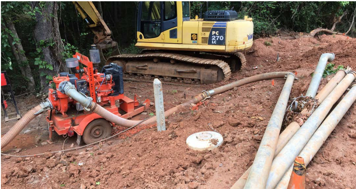
Photo 2: The 12" waterline valve box with collar and marker has been installed at both water connections.
