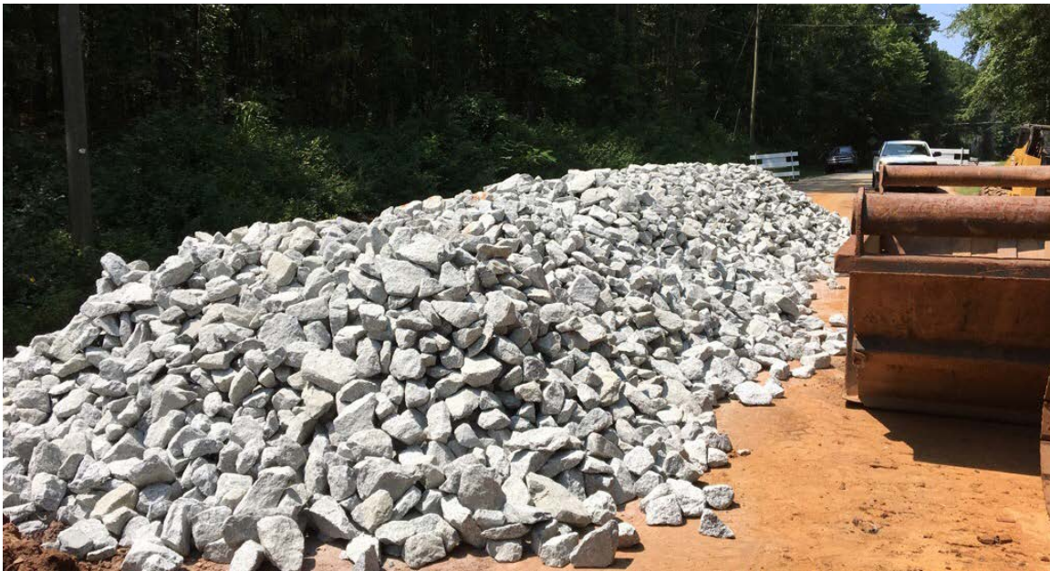
Photo 2: Riprap delivered for upcoming placement at culvert inlet and outlet.
