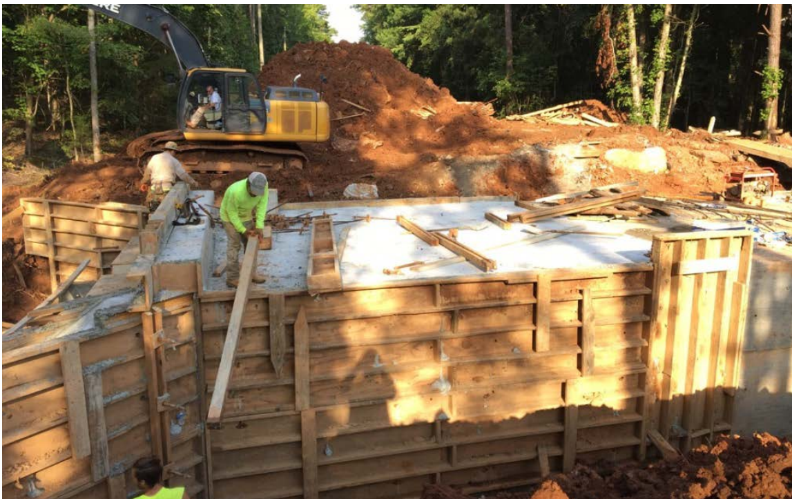
Photo 2: Concrete has been placed for second half of culvert walls, top, and wing walls. Forms are being removed.
