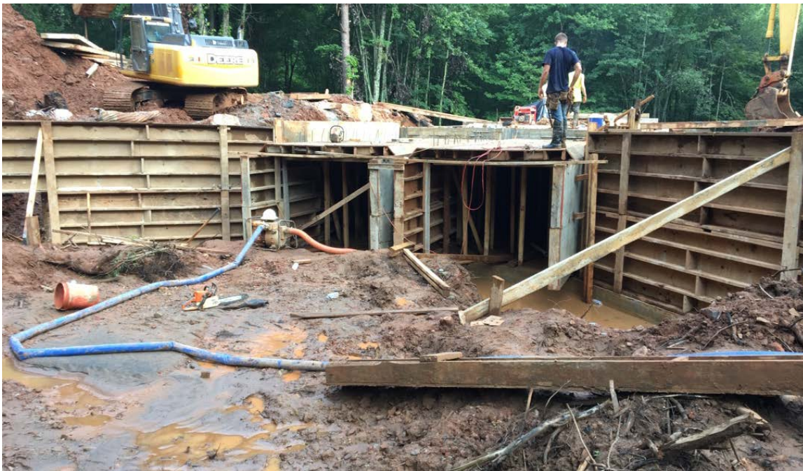
Photo 2: Continue constructing forms and placing rebar for second half of culvert walls, top, and wing walls.
