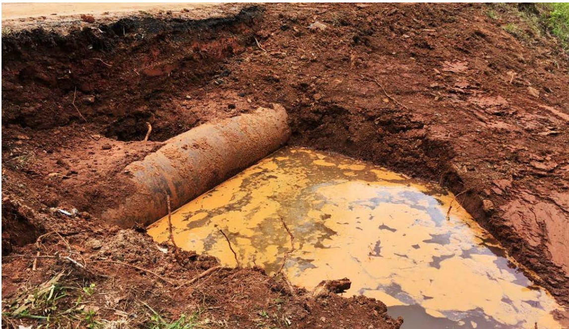
Photo 2: Existing 24" raw waterline running along the north side of Rising Star Road. The line has been exposed and will be relocated soon.
