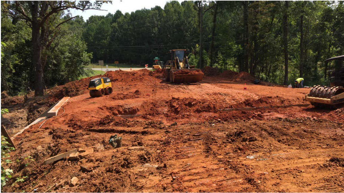
Photo 1: Backfilling and compaction continues. Compaction test completed.
