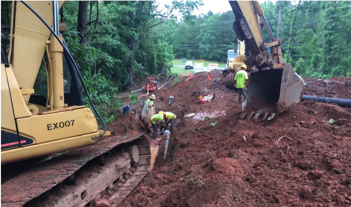
Photo 1: Installation of the 12" waterline.
