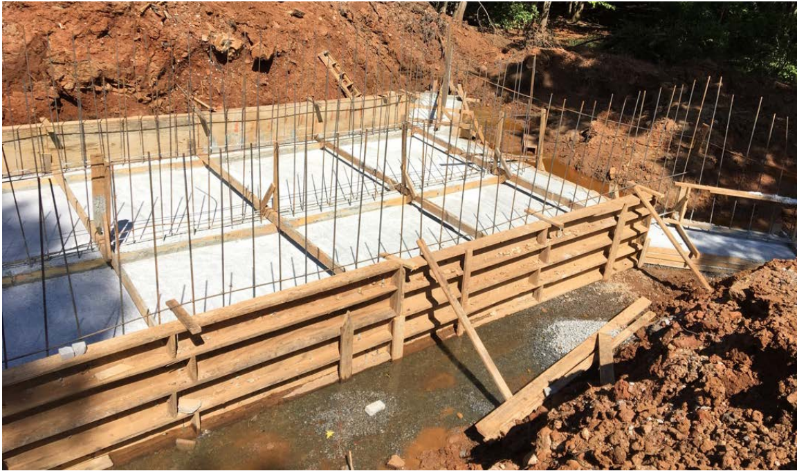
Photo 1: Concrete has been placed for 32 ft. of the culvert bottom slab.
