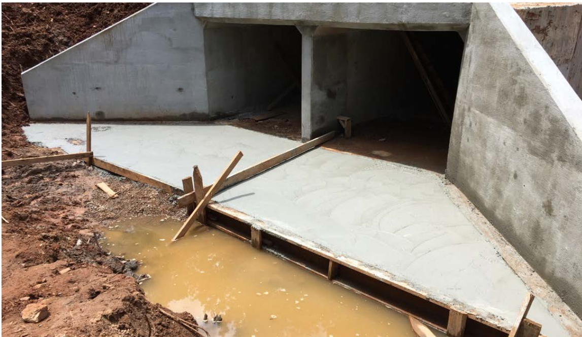
Photo 2: Apron at culvert outlet has been constructed and concrete placed.
