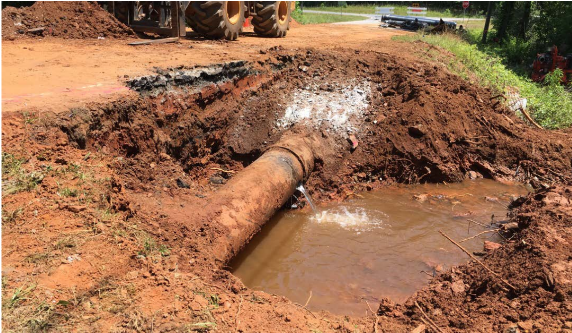
Photo 1: Existing 24" waterline pipe is being drained. (05/09/2018)
