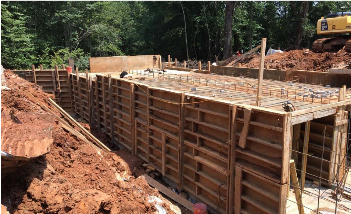
Photo 1: Construction continues on the forms for the culvert walls, top and wing walls.
