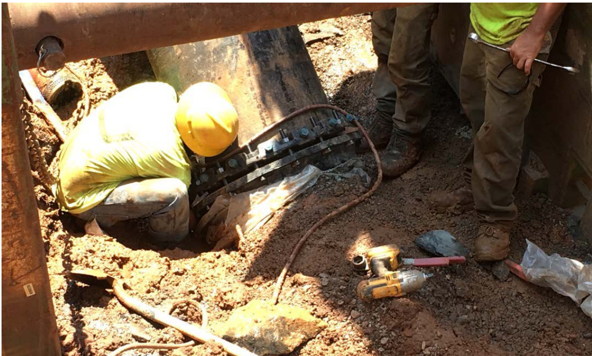
Photo 2: The contactor is installing the 24" waterline pipe and pipe flange.
