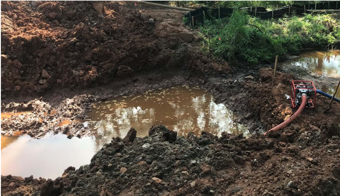
Photo 1: Pooled water continues to be pumped from excavated area. (06/20/2018)
