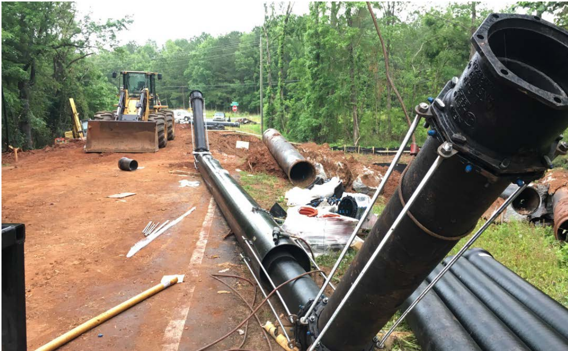
Photo 2: The 12" waterline is ready for installation.
