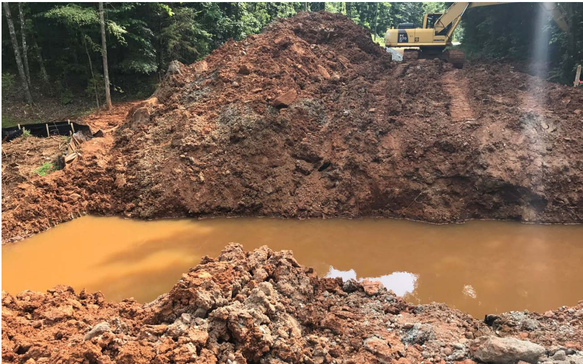
Photo 2: Recent storm events continue to bring excessive water into excavated area. Water must be pumped to allow construction to continue. (06/18/2018)
