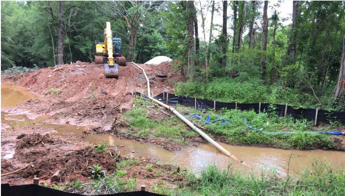
Photo 1: Water diversion has begun at project location. A dam has been built in the creek and water is being pumped over Rising Star Road to the downstream side of the creek.
