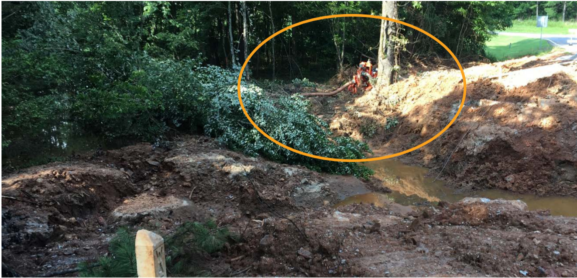
Photo 1: Pooled water continues to be pumped from excavated area.
