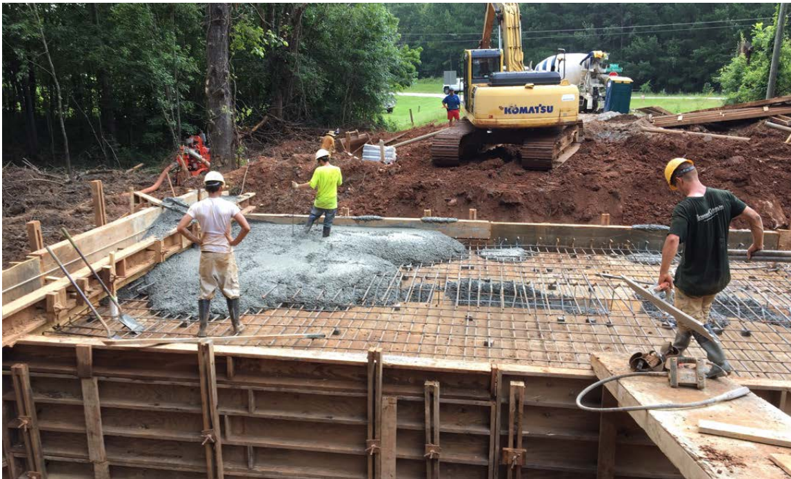
Photo 1: Concrete pouring for the first half of culvert walls and top.
