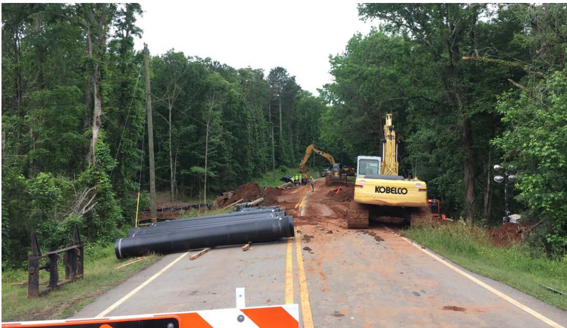
Photo 2: Soil and debris is being removed from road after 12" pipe installation. (05/17/2018)
