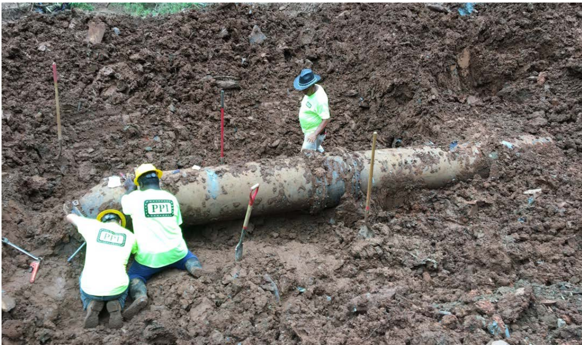
Photo 2: Rod installation at 24" waterline.
