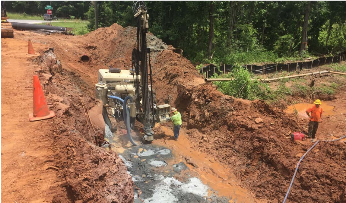
Photo 1: During excavation in mid-May, rock was discovered beneath the existing 24" Raw waterline on the downstream end. The County explored more time-conservative options prior to approving blasting, however other options required additional time and money. Blasting was scheduled and completed as promptly as time allowed. On June 5, 2018, the blasting company was on site and rock blasting was completed.
