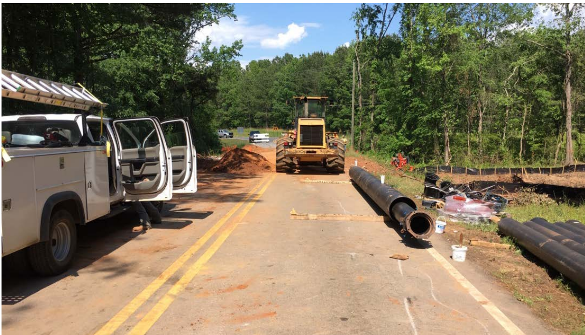
Photo 2: The new 12" waterline pipe and casing is on site and existing pipe is being excavated. (05/08/2018)
