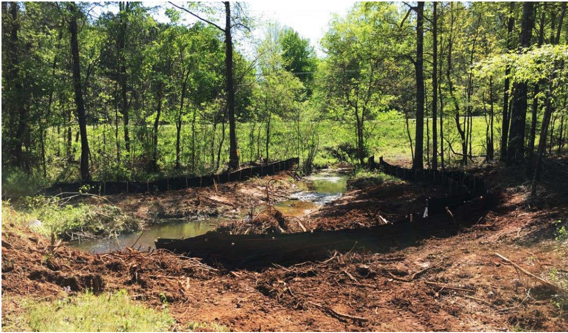
Photo 1: Double row silt fence installed near creek for erosion control.
