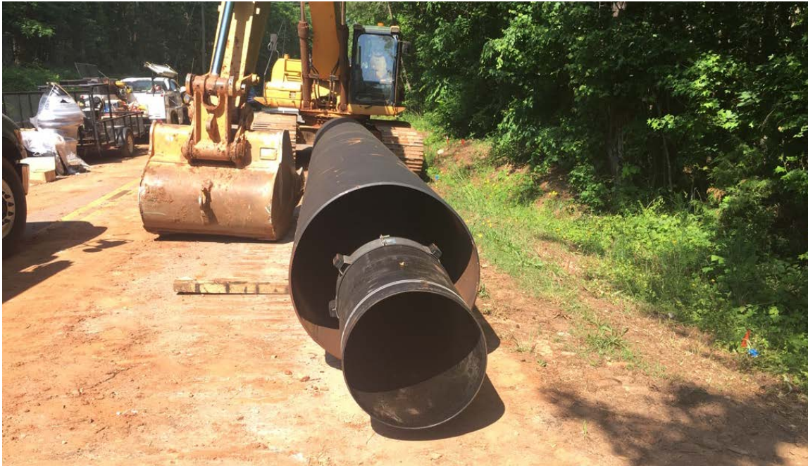
Photo 1: Preparing 24" waterline for installation.
