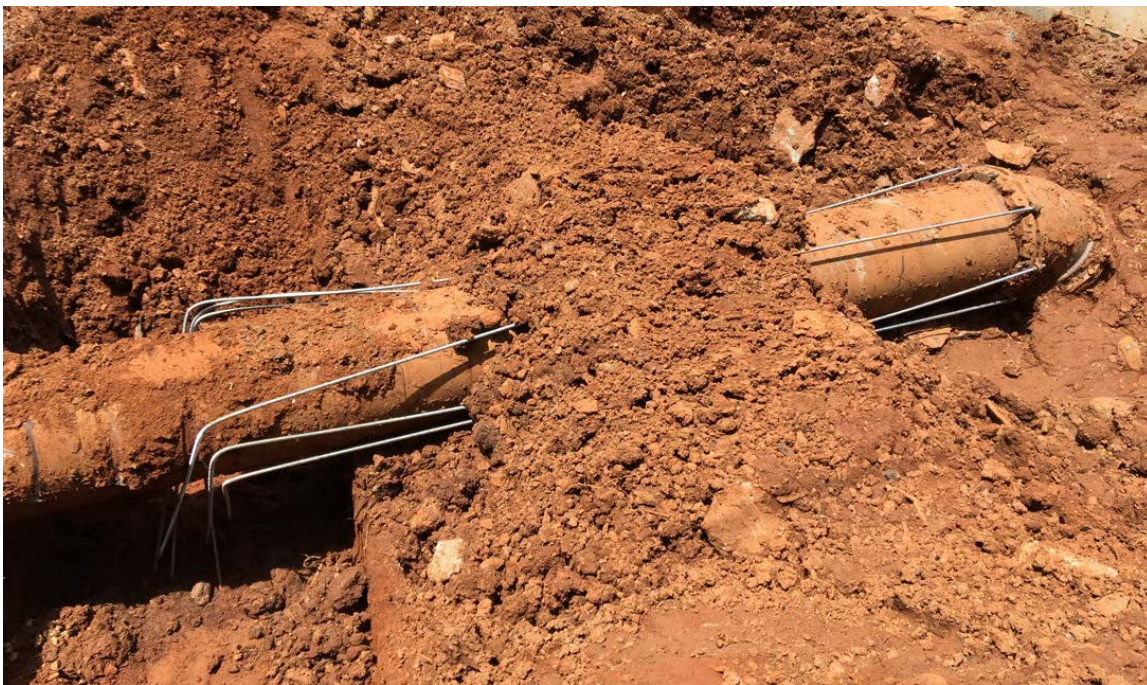
Photo 2: Rod installation is complete. The area for 24" waterline concrete blocking has been excavated.
