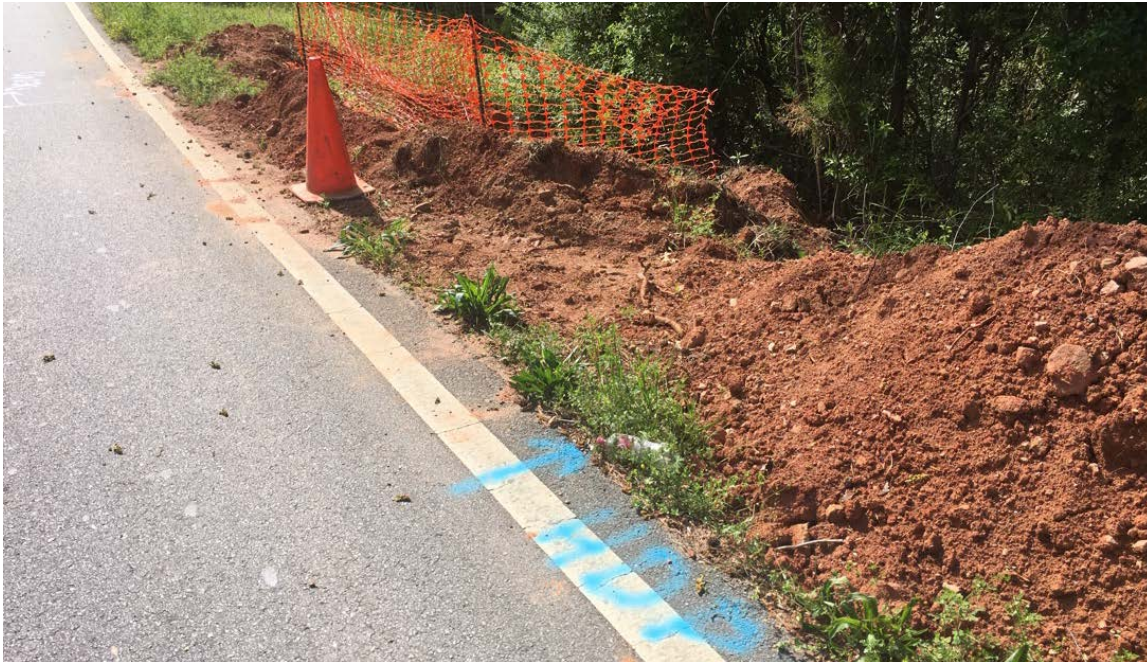
Photo 1: Utility relocation has begun. The utilities at the project site have been located, marked, and excavated.
