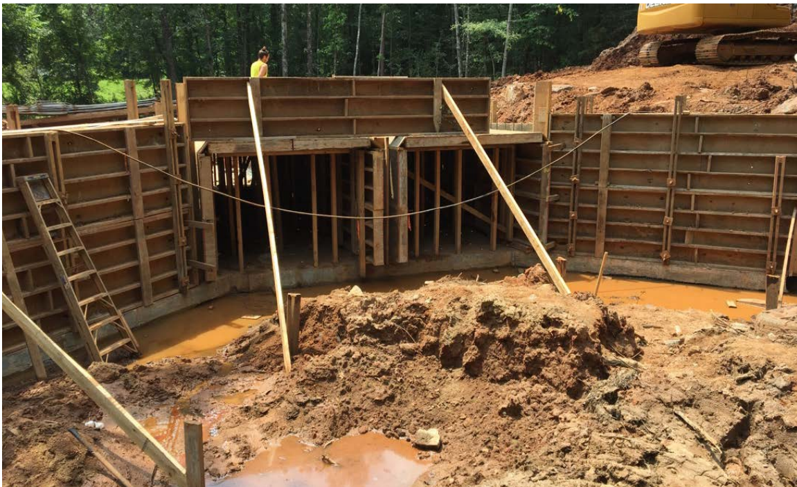
Photo 2: Construction continues on the forms for the culvert walls, top and wing walls.
