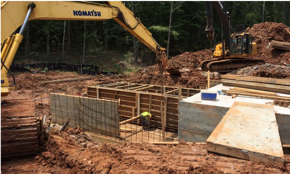
Photo 2: Constructing forms for the second half of culvert walls, top, and wing walls.
