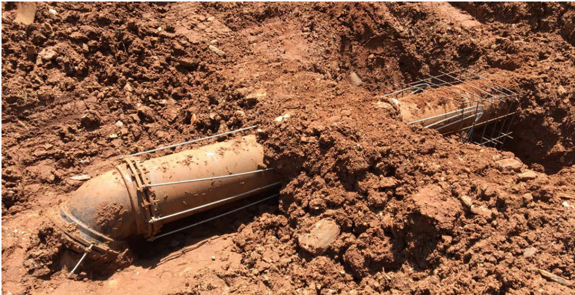
Photo 2: Rebar has been placed around the waterline for the concrete block.
