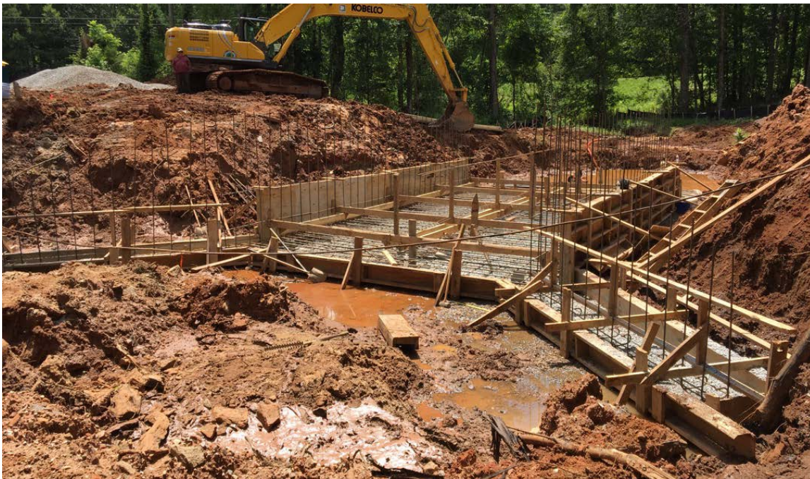
Photo 2: Forms and rebar for the upstream wing walls of the culvert bottom slab have been placed. Concrete is expected to be poured today.
