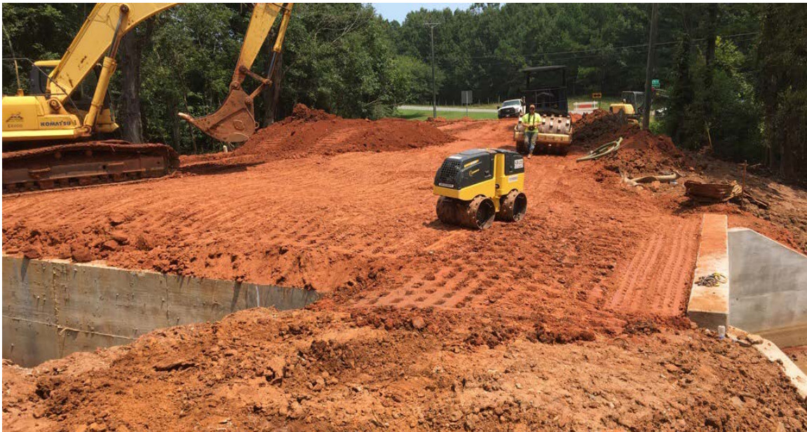
Photo 2: Backfilling and compaction in progress.
