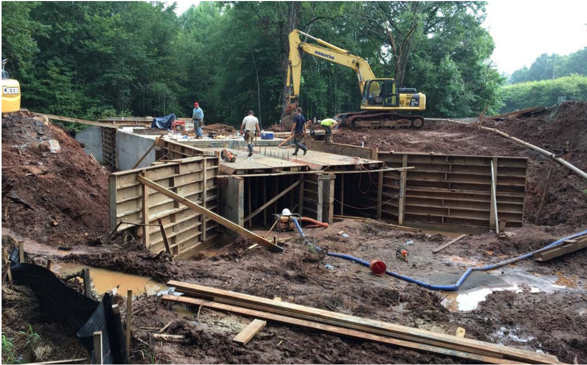
Photo 1: Continue constructing forms and placing rebar for second half of culvert walls, top, and wing walls.
