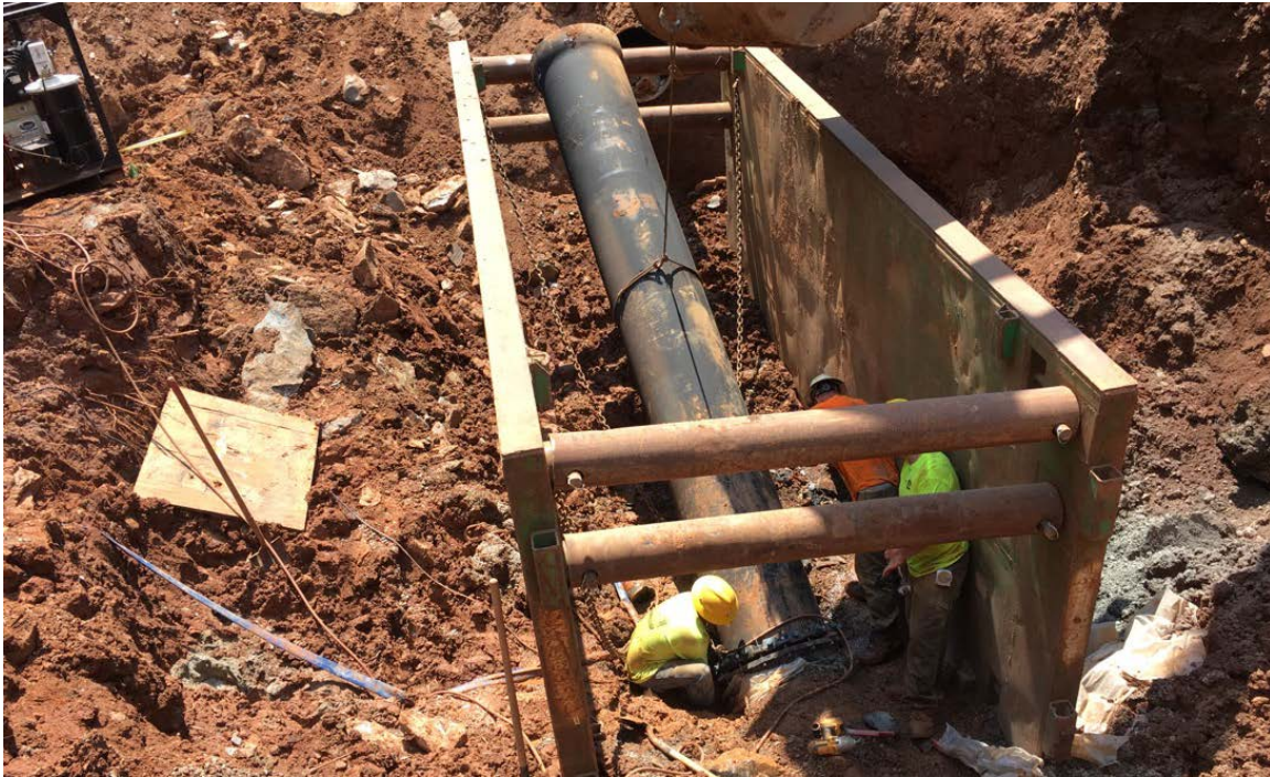
Photo 1: The contactor is installing the 24" waterline pipe and pipe flange.
