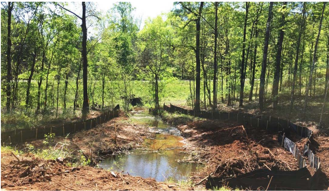
Photo 2: Double row silt fence installed near creek for erosion control.
