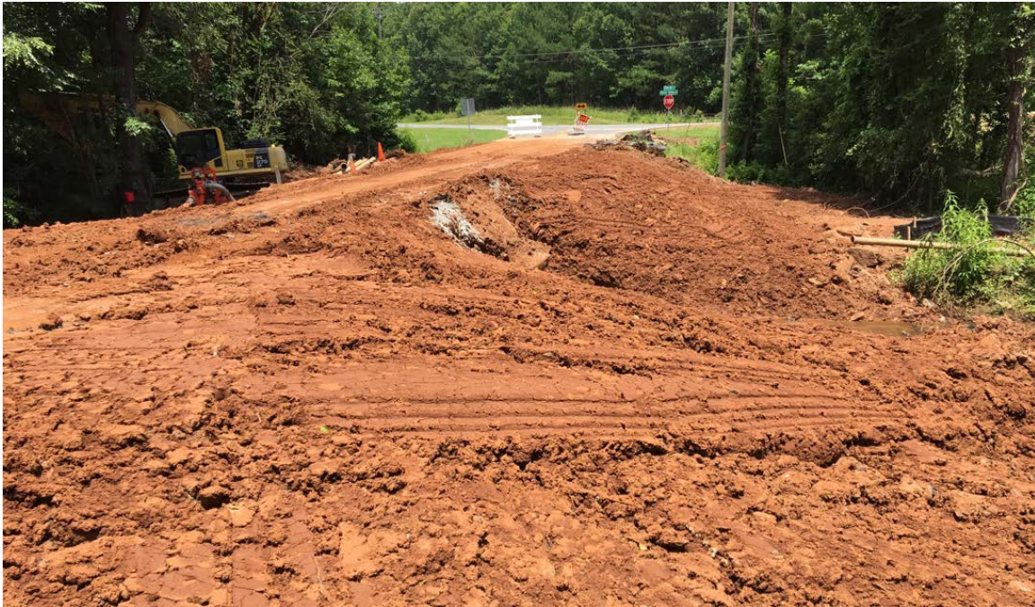
Photo 1: The 24" waterline installation is complete and the trenches have been backfilled.
