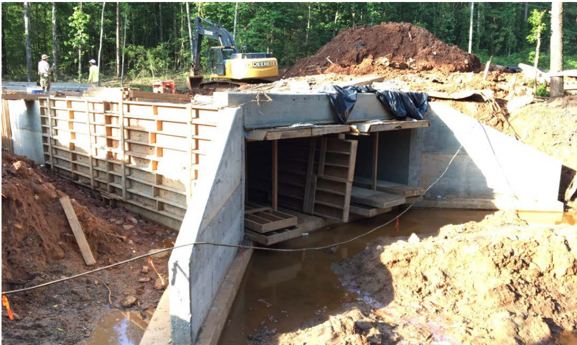
Photo 1: Concrete has been placed for second half of culvert walls, top, and wing walls.
