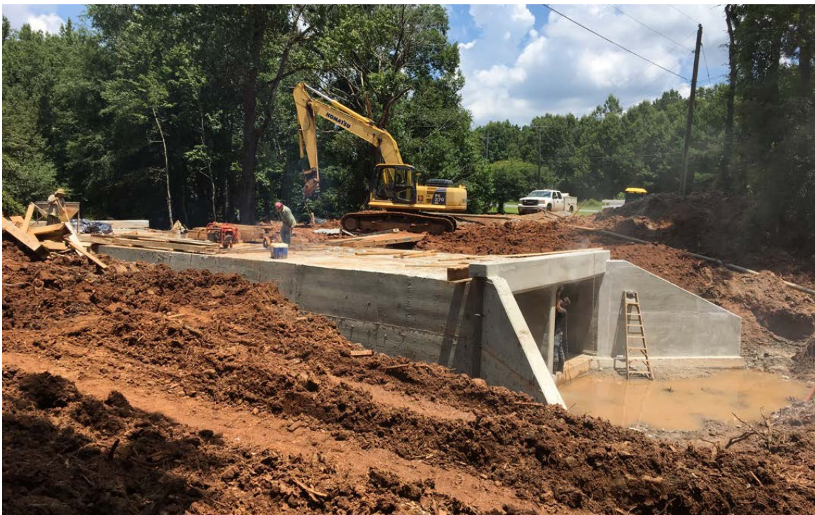
Photo 2: Culvert construction is complete. Site cleaning is underway.
