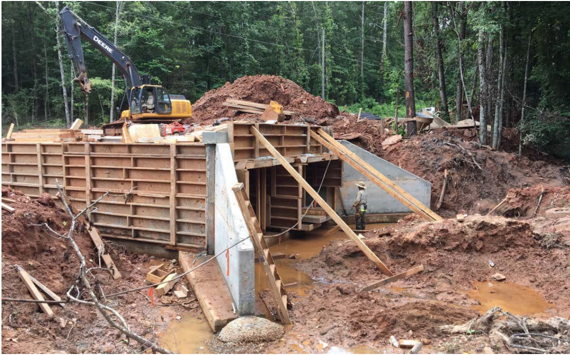
Photo 1: Removing forms from the 07/13/2018 concrete pour on the first half of the culvert.
