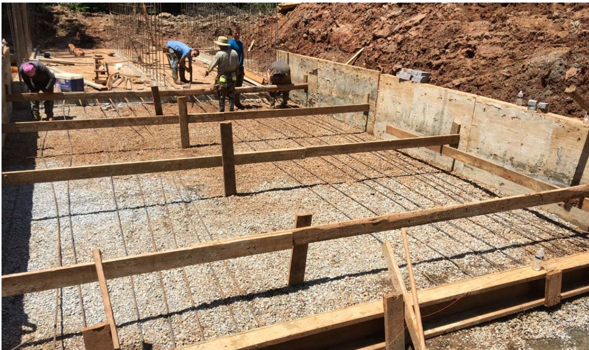
Photo 2: Gravel, forms, and rebar for the second half of culvert base are under construction.
