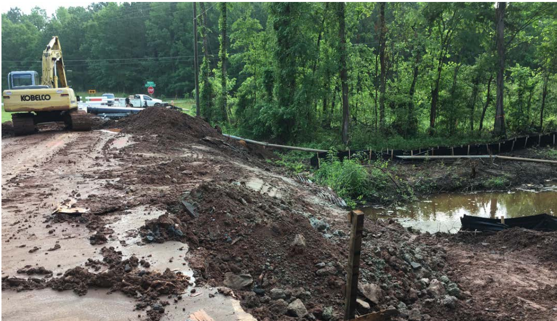
Photo 1: During excavation, rock was located in the area where the 24" waterline is to be installed. Installation is delayed until rock blasting is completed. (05/18/2018)
