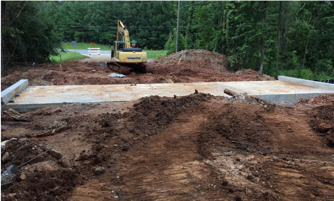
Photo 1: View of completed culvert top.
