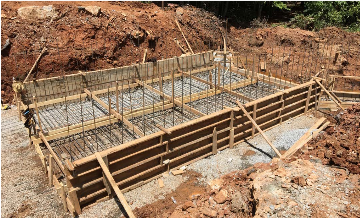
Photo 1: Gravel has been placed in the culvert base. Forms and rebar for 32 ft. on the upstream side of the culvert bottom slab have been placed. Concrete is expected to be poured today.
