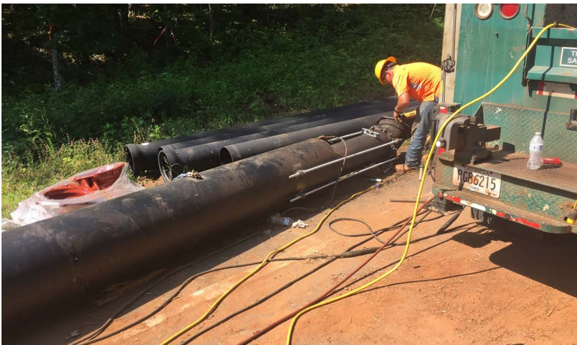
Photo 2: Preparing 12" waterline for installation.
