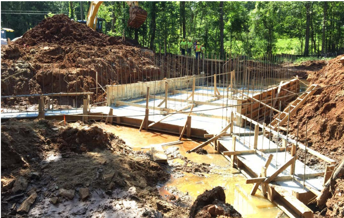
Photo 2: Concrete has been placed for upstream wing wall base.
