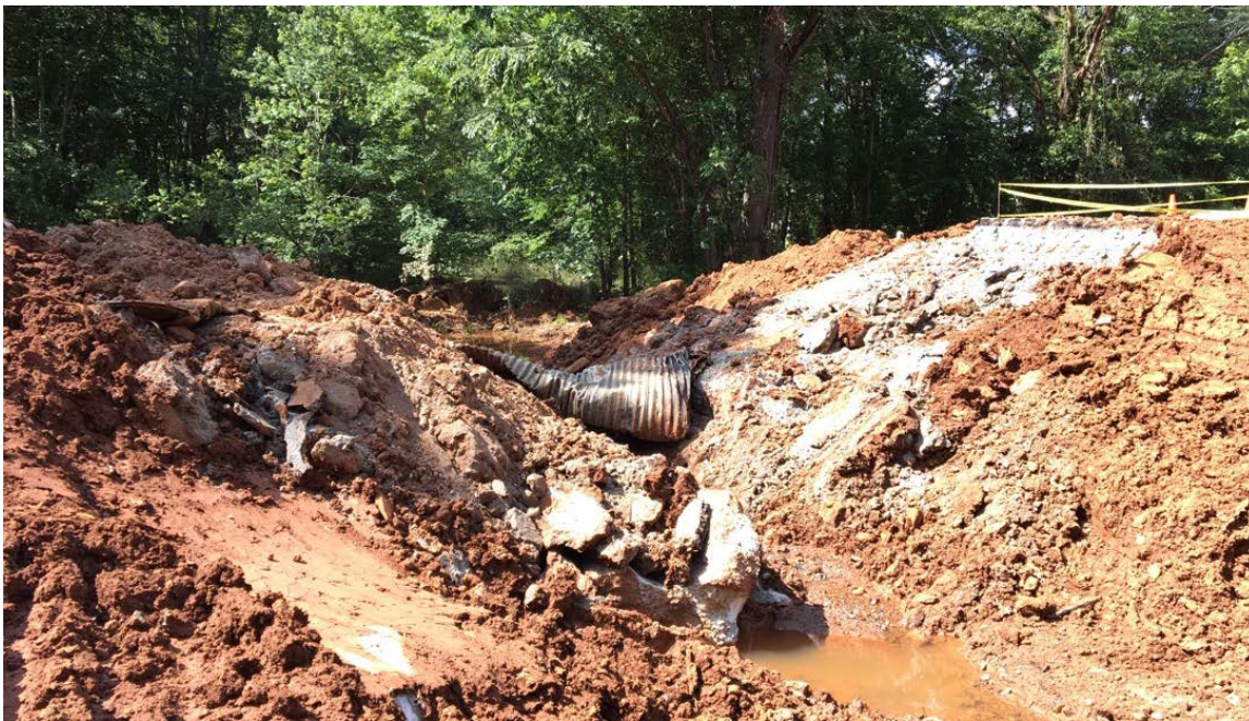
Photo 2: Demolition of existing box culvert and Rising Star Road has begun. (06/13/2018)
