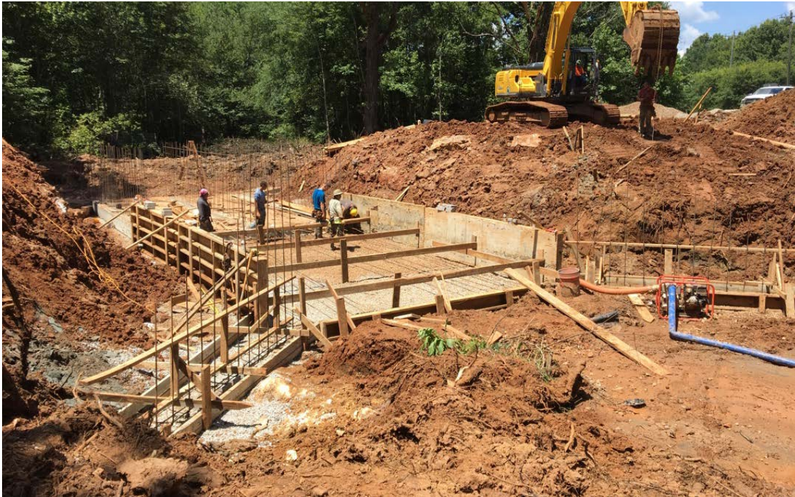
Photo 1: Forms and rebar for the second half of culvert base and wing wall base are under construction.
