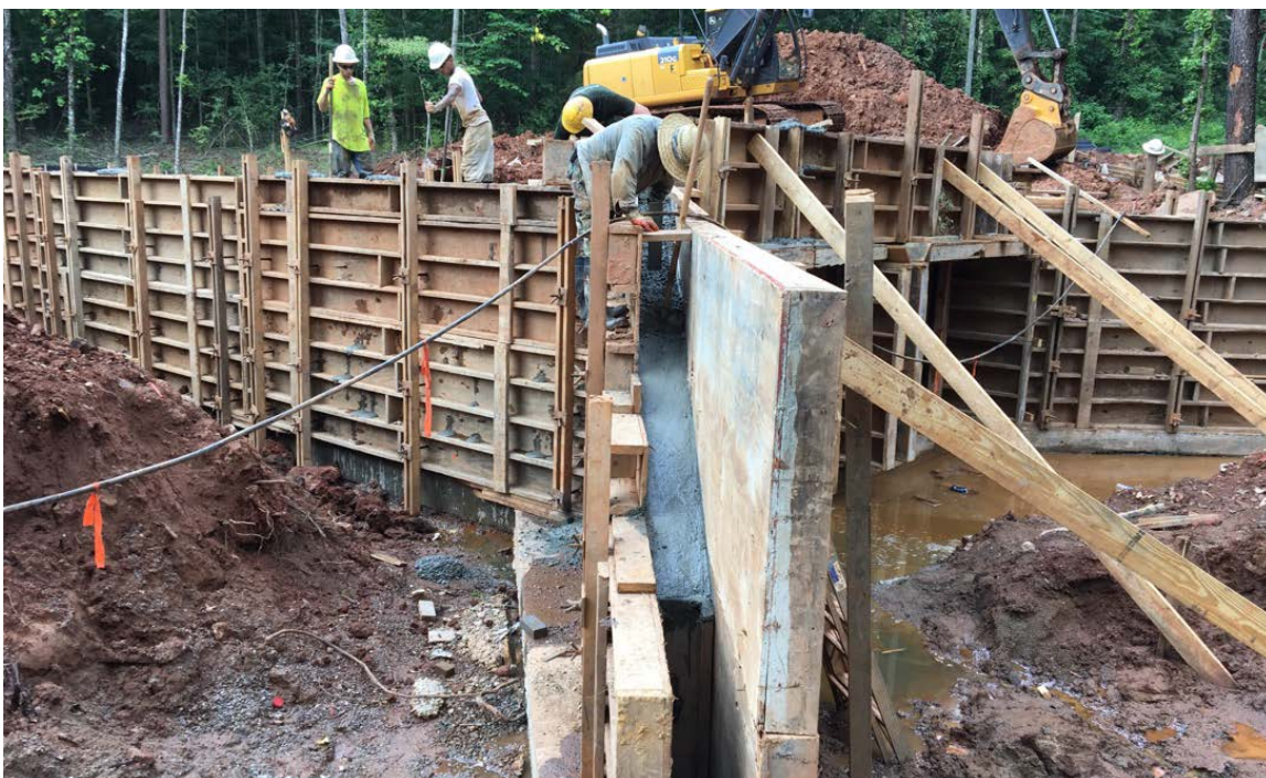
Photo 2: Concrete pouring for the first half of culvert wing walls.
