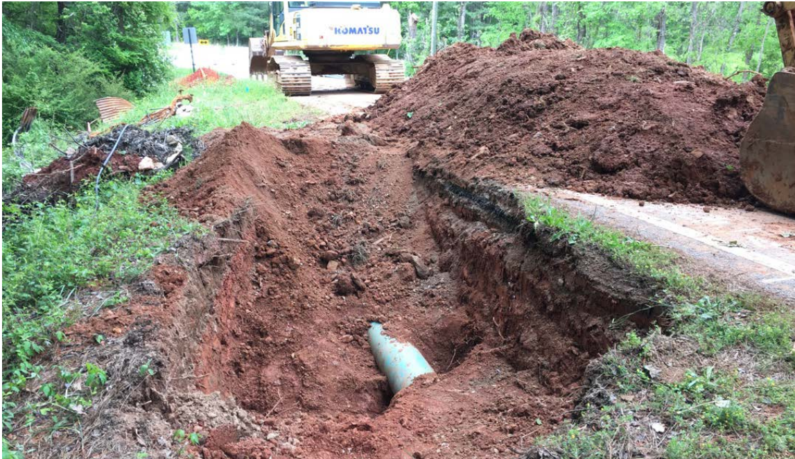
Photo 1: Existing 12" potable waterline running along the south side of Rising Star Road. The line has been exposed and will be relocated soon.
