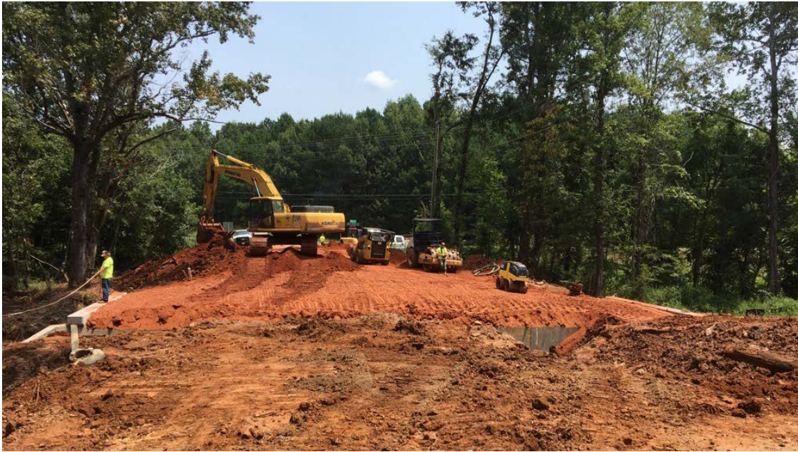
Photo 1: Backfilling and compaction in progress.
