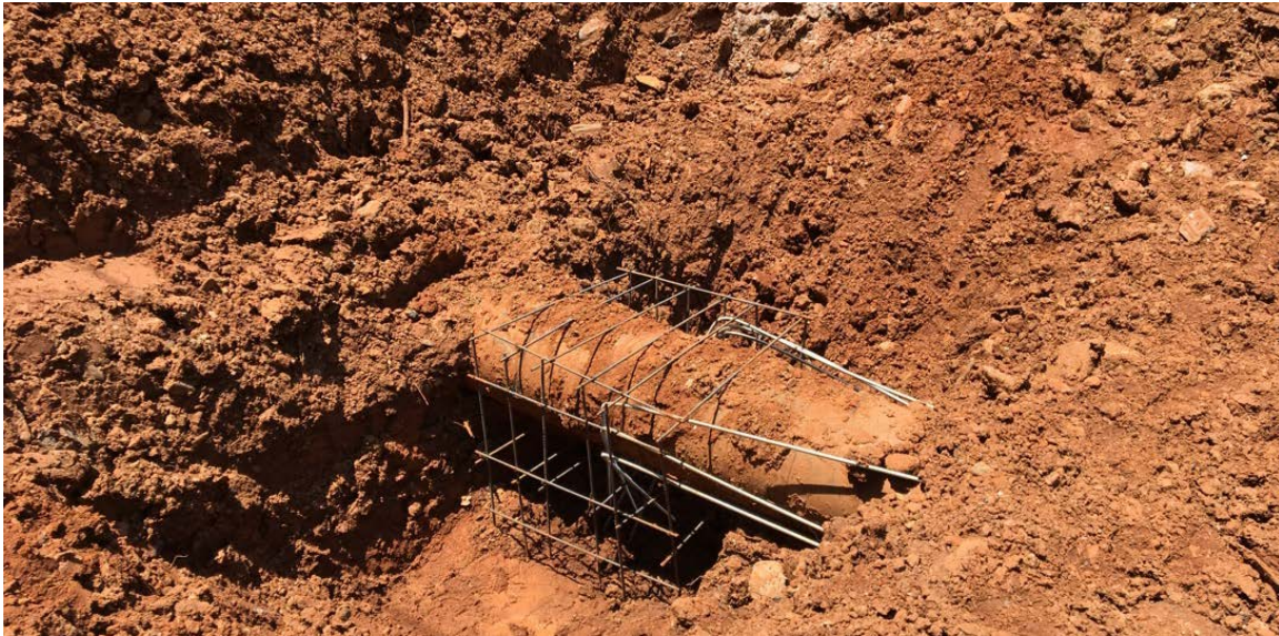
Photo 1: Rebar has been placed in the void around the waterline for the concrete block.
