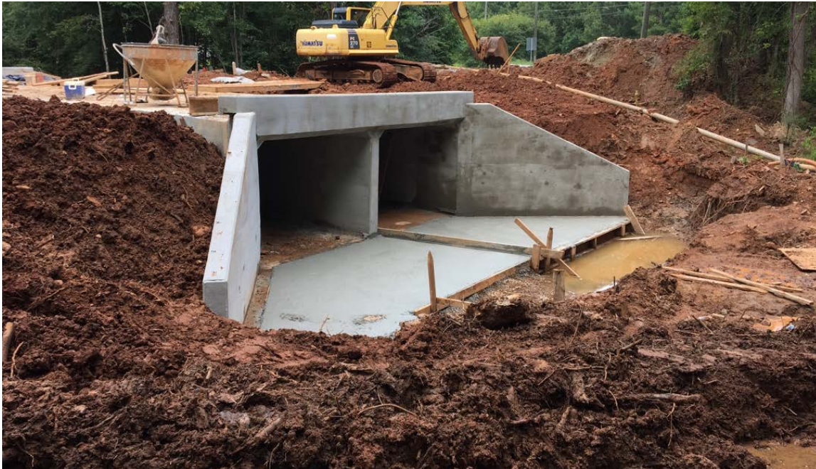
Photo 1: Apron at culvert outlet has been constructed and concrete placed.
