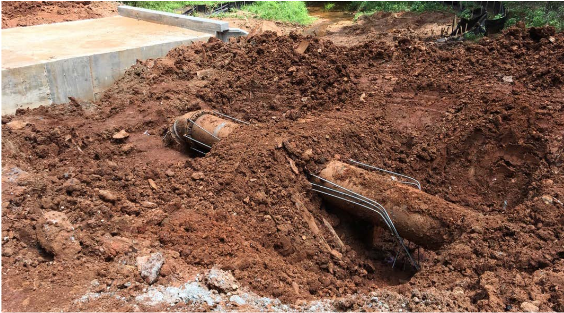
Photo 1: Rod installation is complete. The area for 24" waterline concrete blocking has been excavated.
