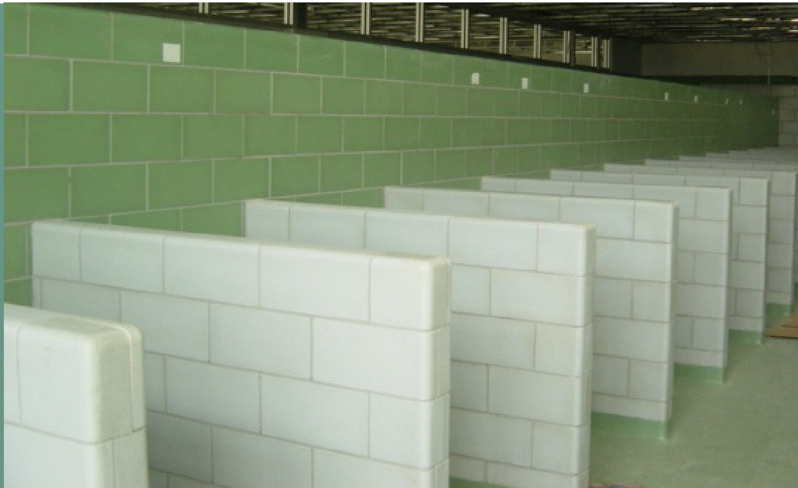
Interior Kennel Space Material - GLAZED CMU New kennels could be constructed using glazed CMU, which is easier to clean, resulting in a more hygienic space.
