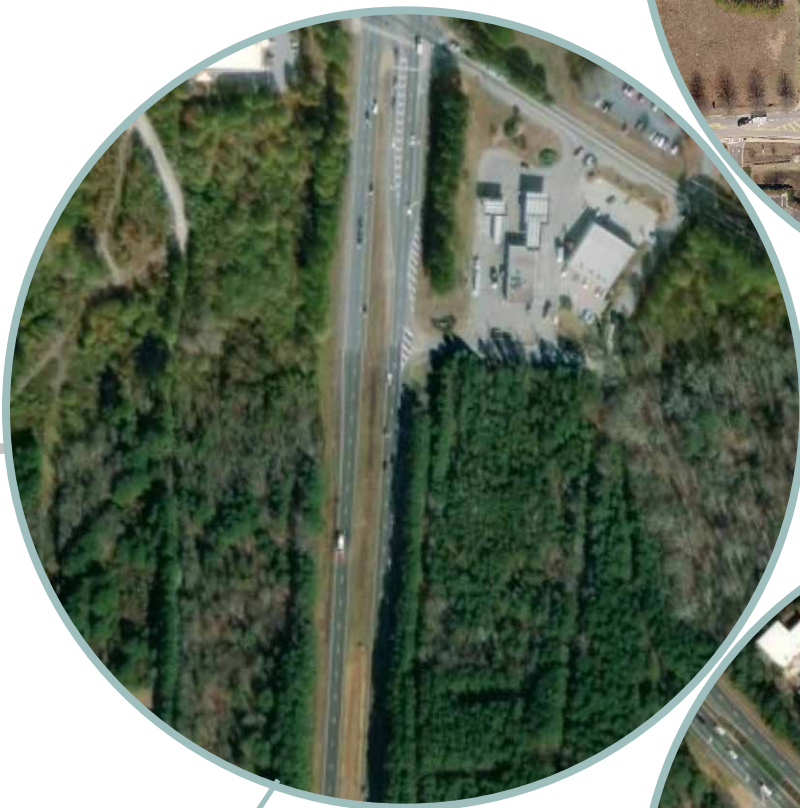
In the Tyrone area, much of the corridor has a rural feel and bicycle and pedestrian facilities are not common
