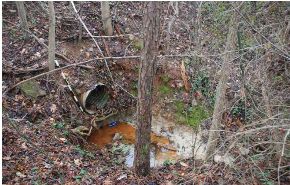
Photo 2: Downstream end of culvert.
