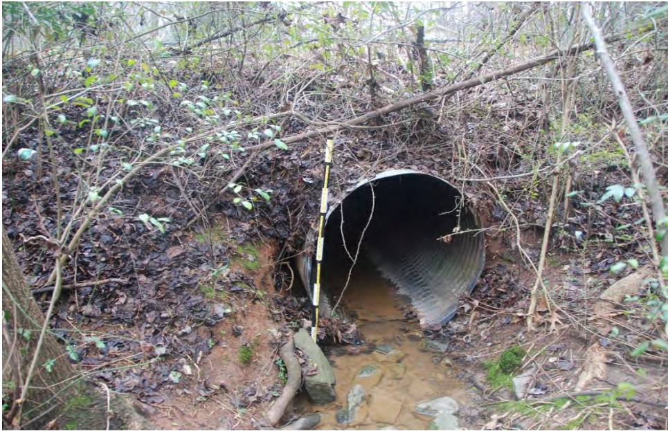
Photo 1: Upstream end of culvert.
