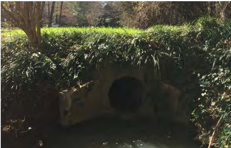
Photo 2: Downstream end looking West towards Deauville Way.
