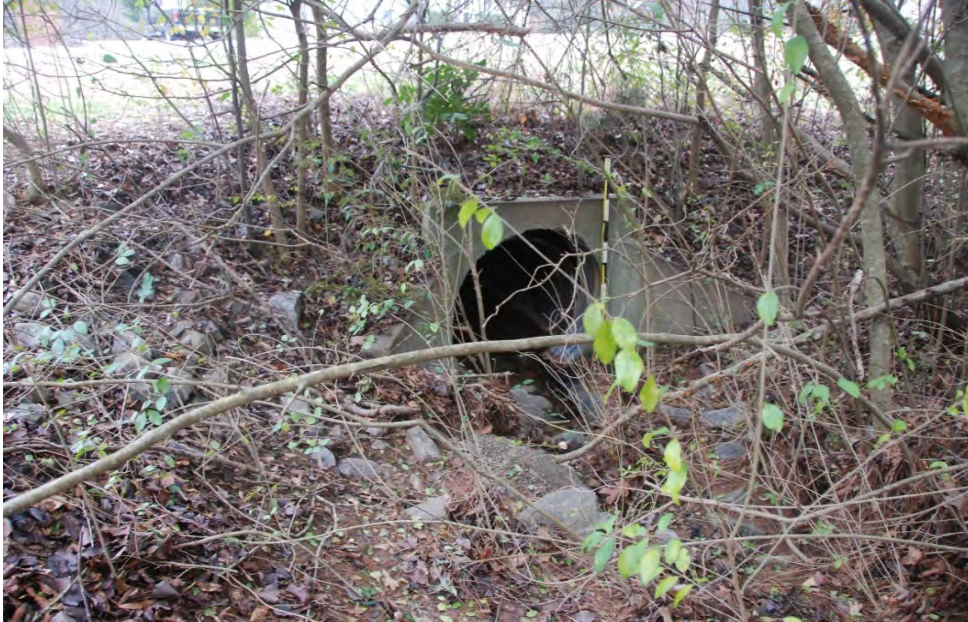
Photo 1: Upstream end of culvert.
