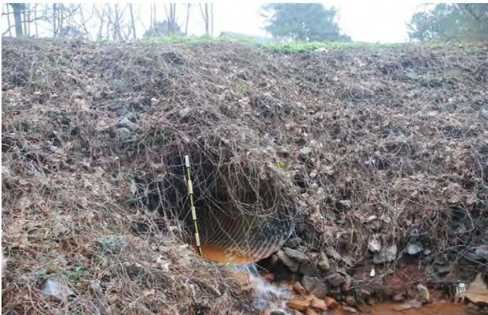
Photo 2: Downstream end of culvert.
