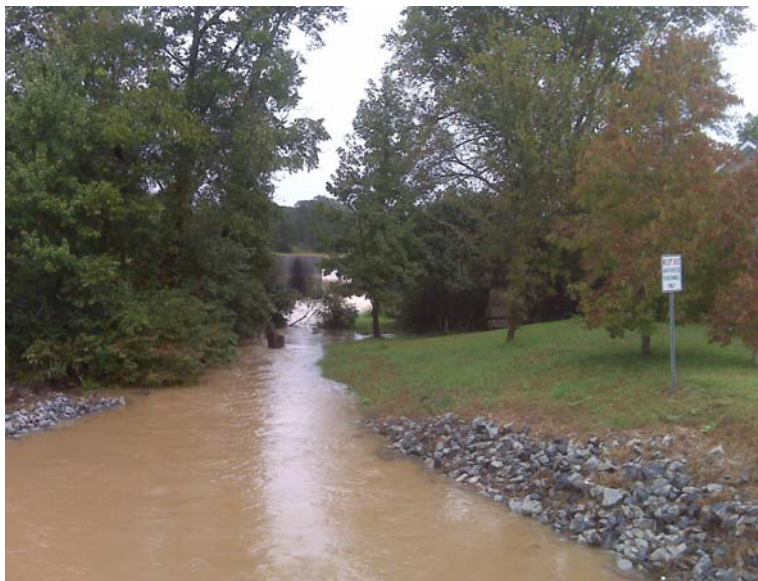
Completed Pye Lake Hazard Mitigation Drainage Project
