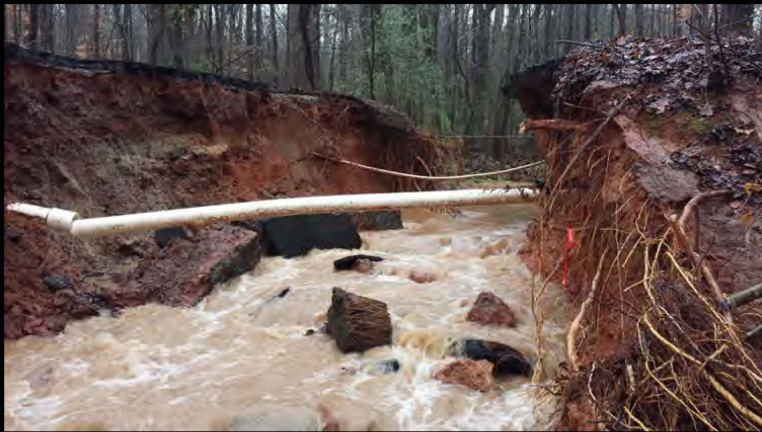
Looking upstream; broken water line in foreground, gas line in background
