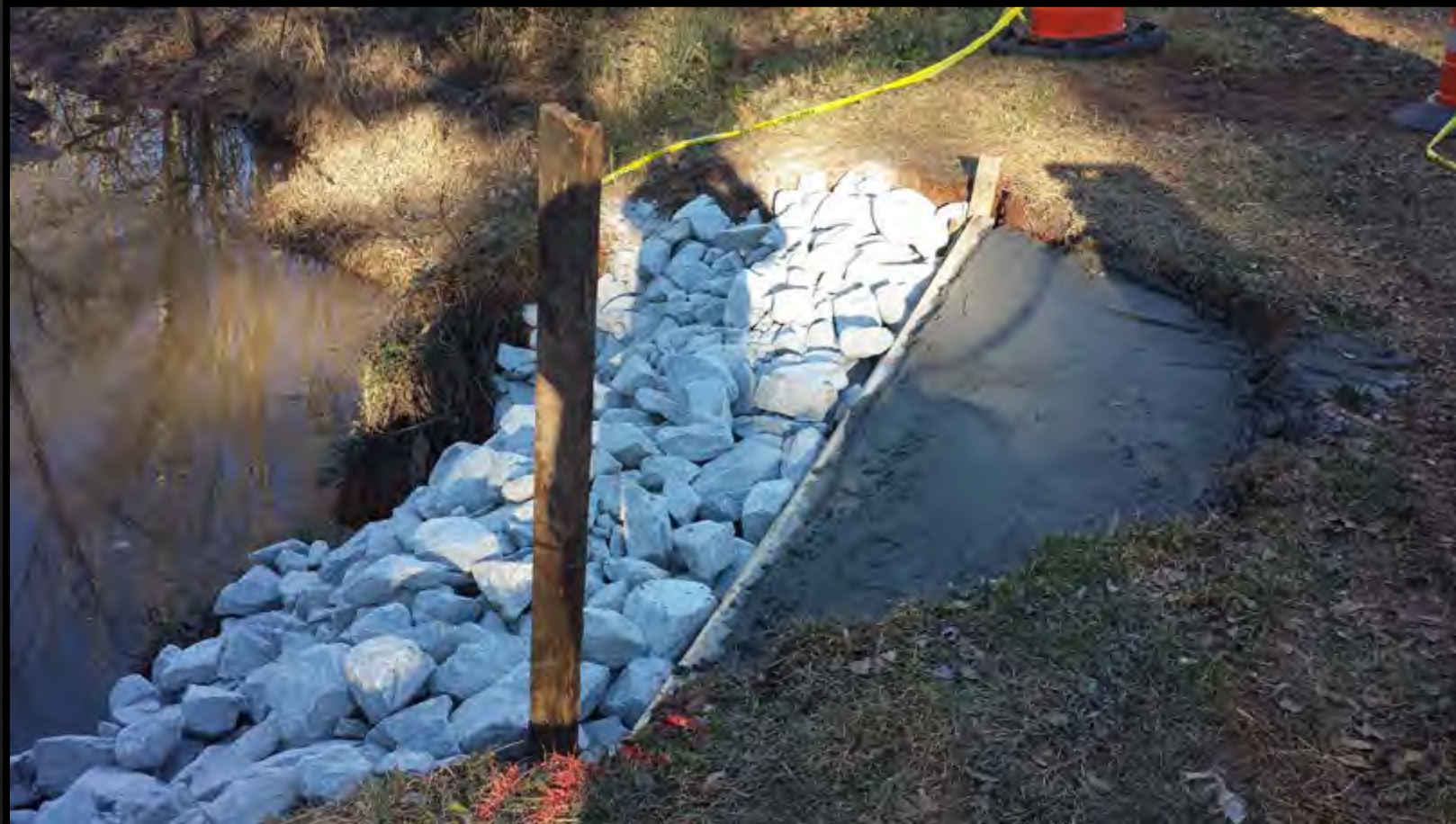
Flowable Fill poured January 5th
