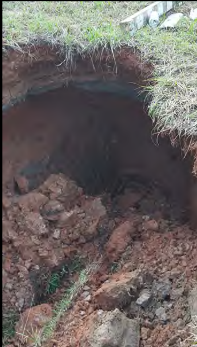
Washout around pipe – December 25 th
