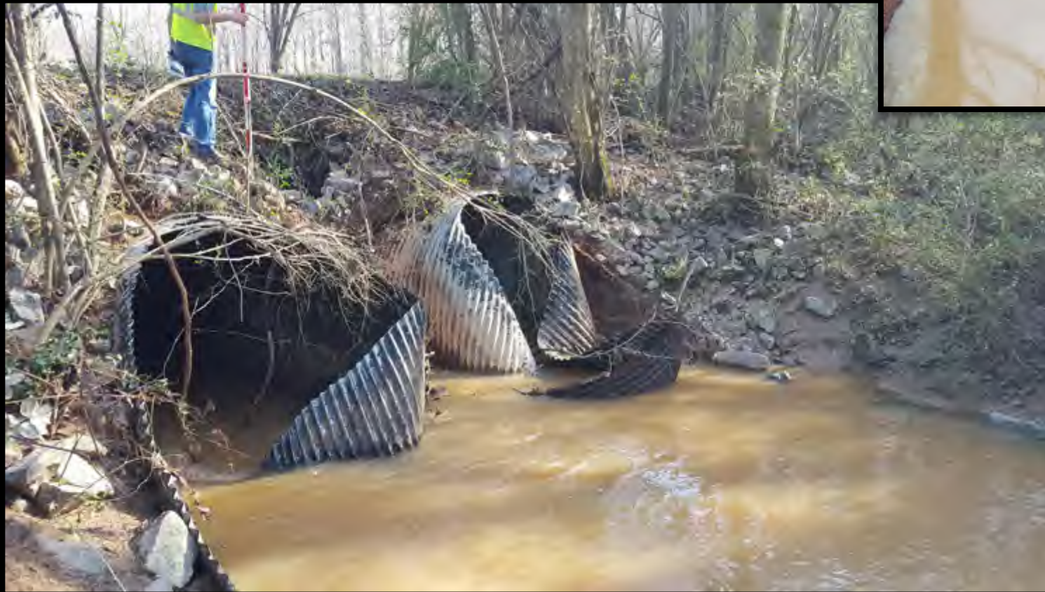
Upstream Pipe Inlets December 29 th
