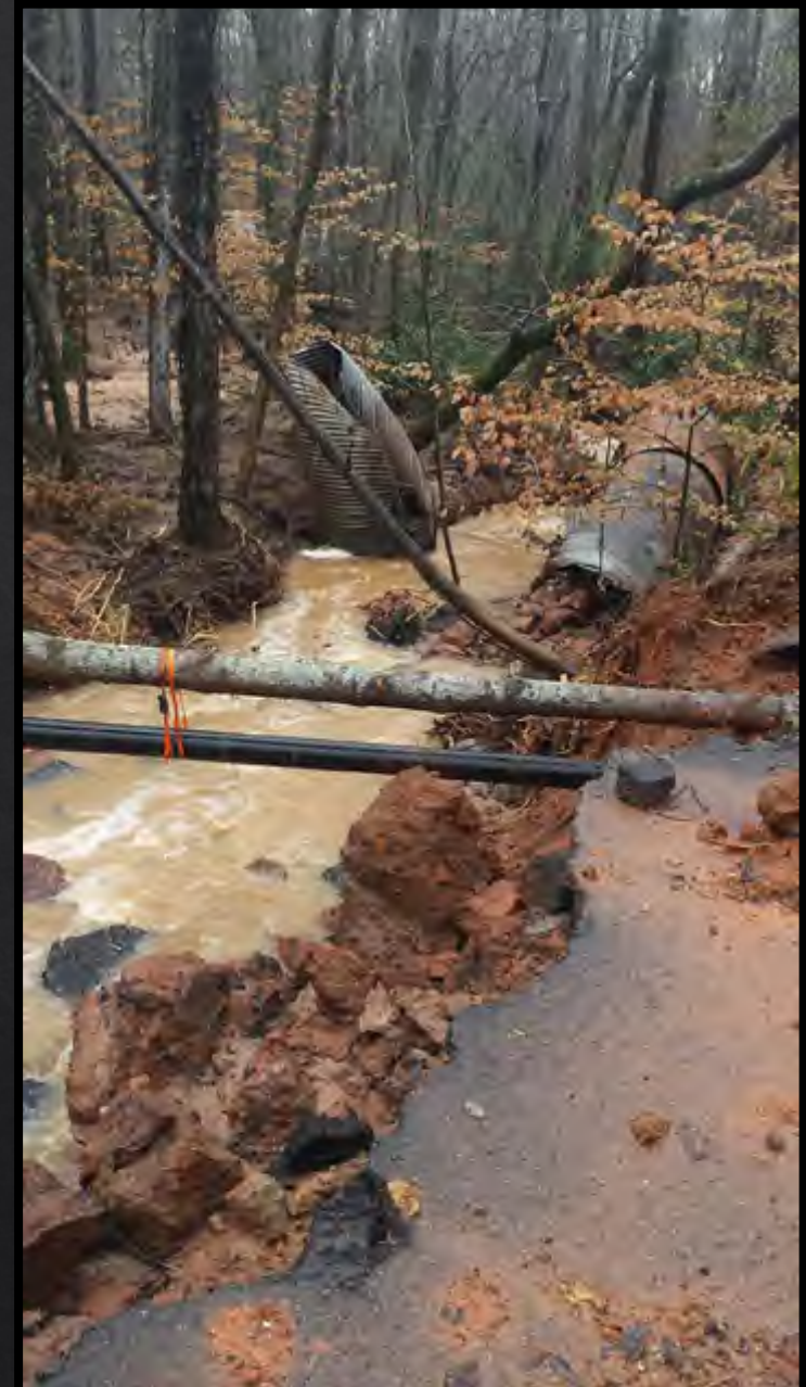
Looking downstream; new waterline installed Christmas Eve
